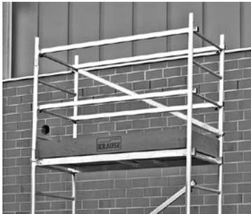
This picture shows the completely mounted side protection.
