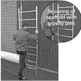
Securing of scaffold with gravity pins
