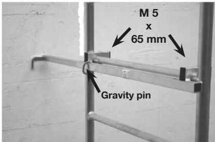
Mount the set of stabilisers to the wall by using a set of stabilisers. The set of stabilisers prevent the scaffolding (mobile working platform) from tilting against the wall. In case of using the sets of stabilisers it is essential to take care that these sets are always mounted below the top platform.
