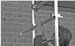
The picture shows how to adjust a stabilizing set.
