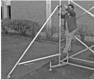
The picture shows an attached outrigger.
